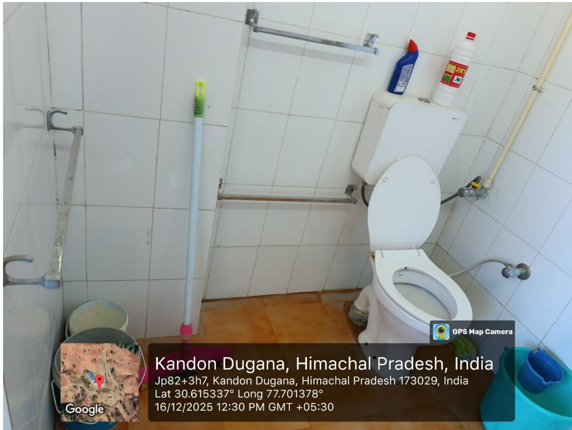
Figure 4: Toilet for Specially abled students (Inside)
